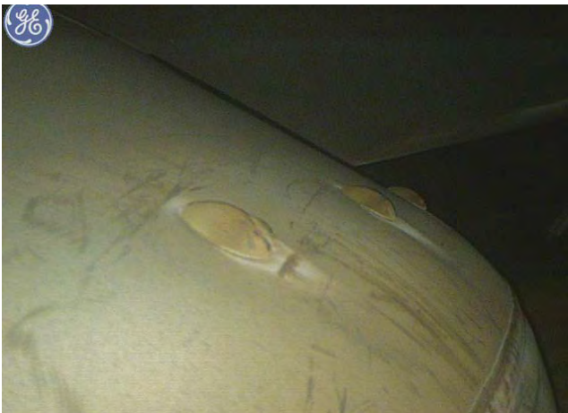
Inner liner rivets and struts.
