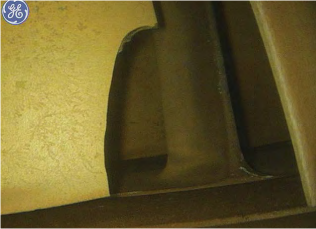
HPC STG12 Blade Missing on T/E side Serviceable Table:4, 2/b
